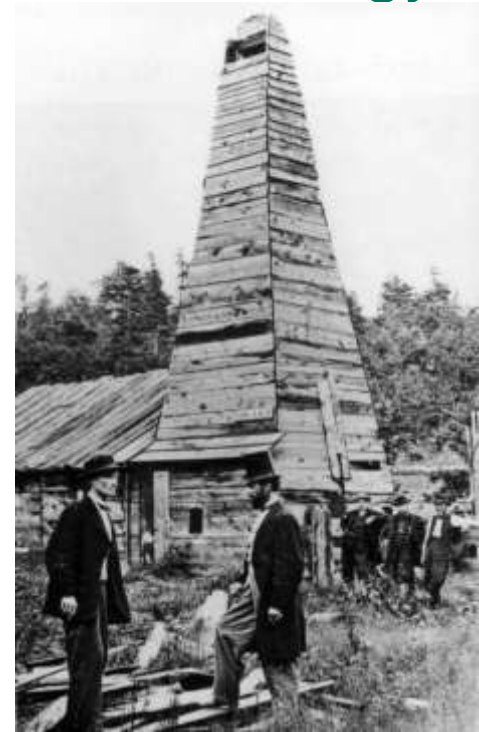
1857 First Oil Well In Pennsylvania
