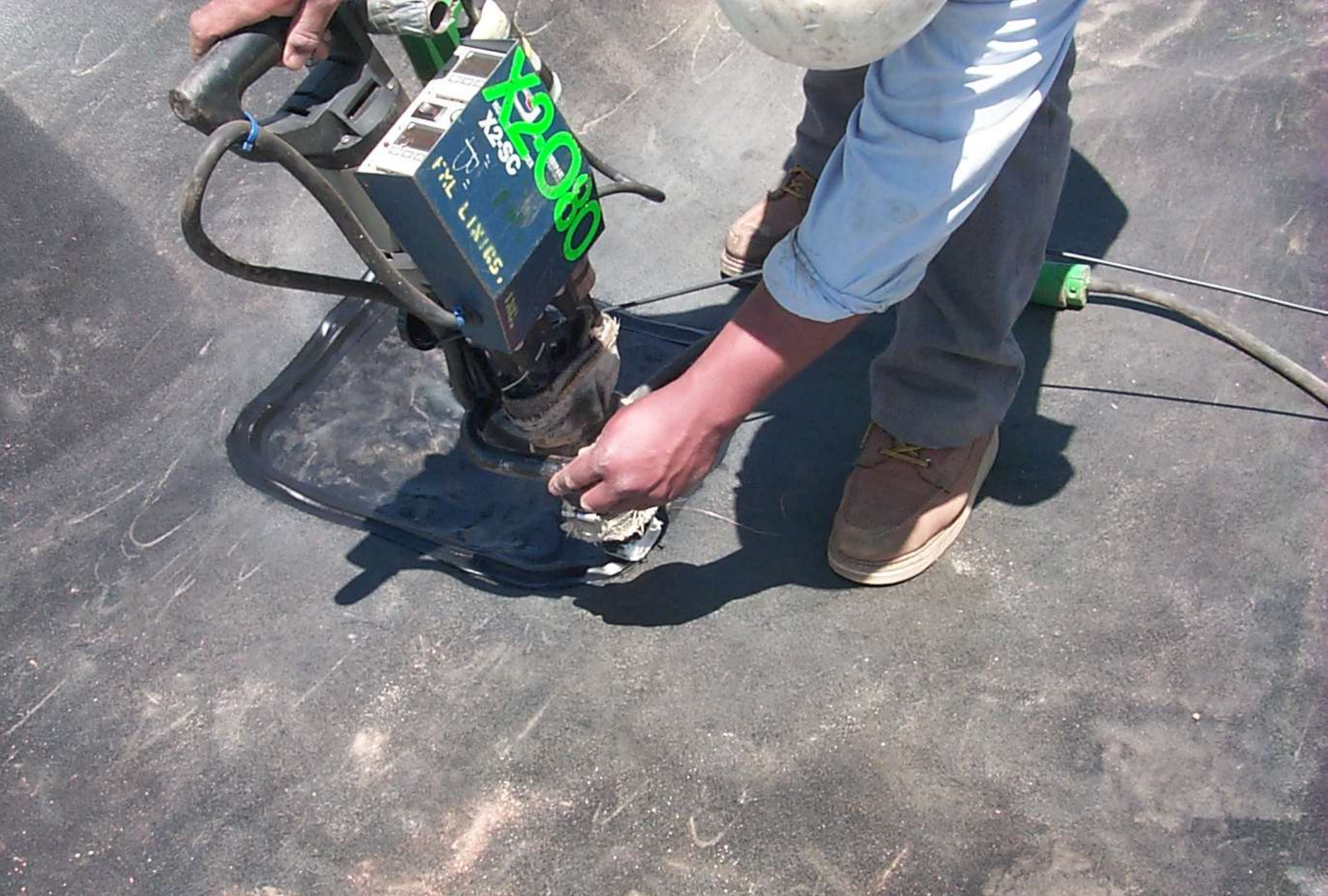
Extrusion welding sump boot.
