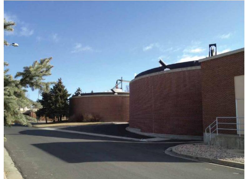
Anaerobic Digesters at Drake Water Reclamation Facility
